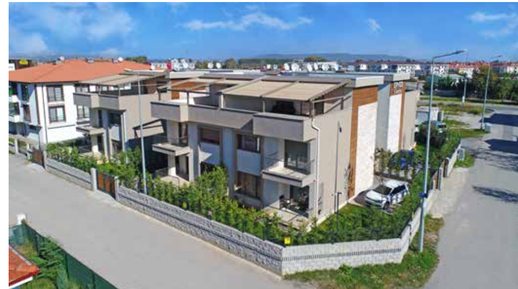
ERVES iGarden Villa Project
